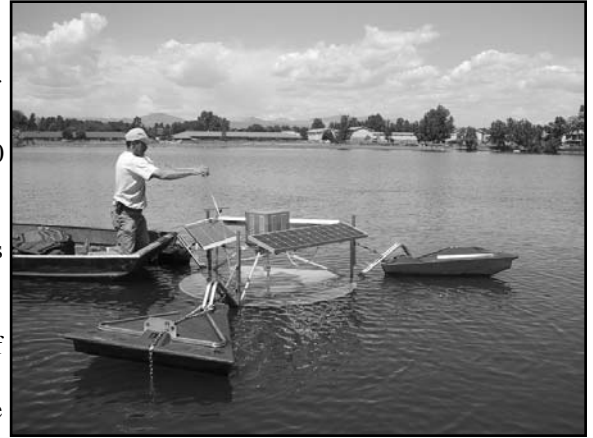
Mike Borsma of Pump Systems, Inc. installs the Solar Bee in Silver Lake.
